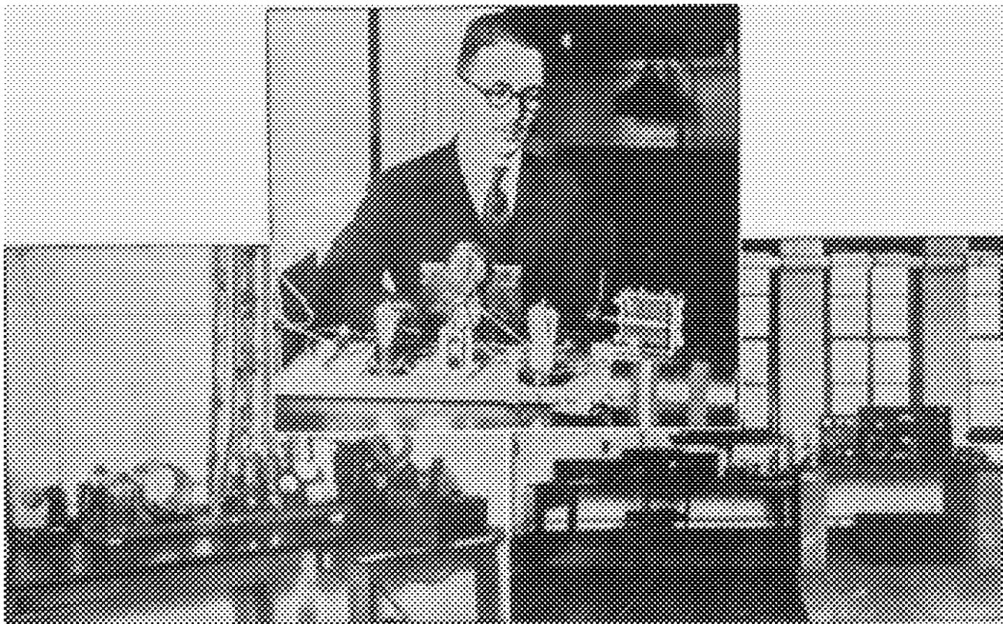
**Center:** Mr. Schnell and his 110 meter receiver. **Lower left:** The 110 meter transmitter at 1MO. **Lower right:** Receiving and broadcasting station at Haverford College, where signals from Leon Delon's amateur station at Nice France were brought in on a loud speaker.
